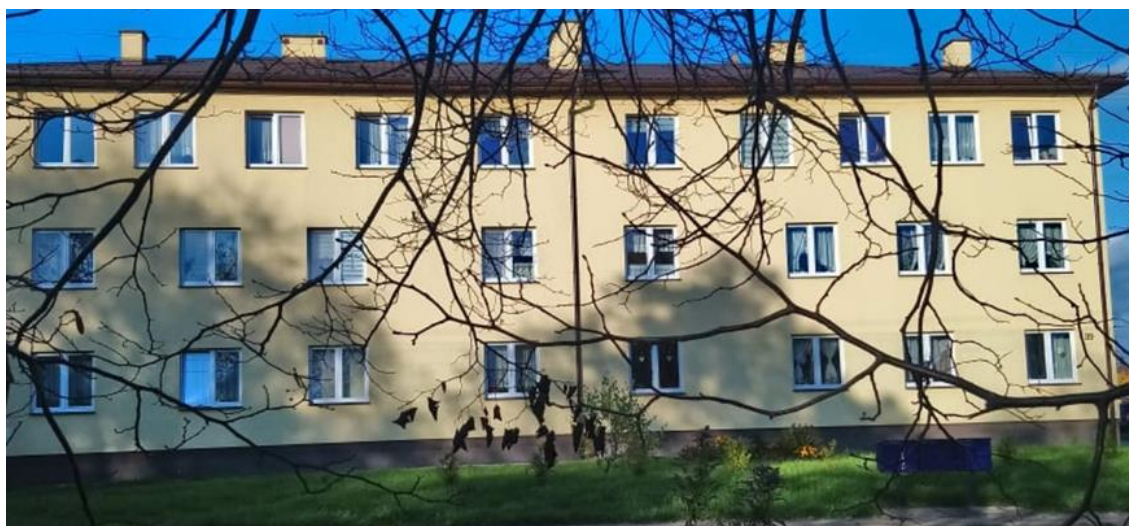
Figure 8-2. Building no. 39 in Maty Klincz (front side)
