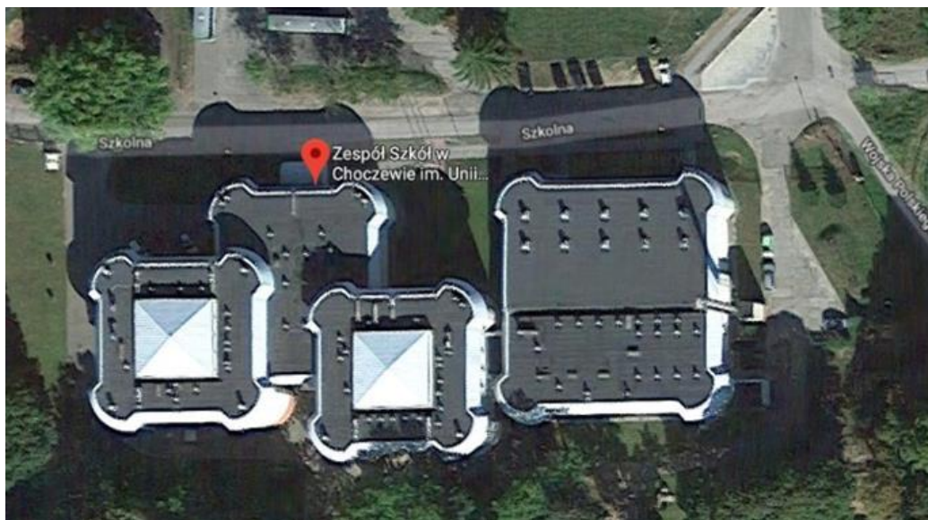
Figure 6-1. Top view of the building
