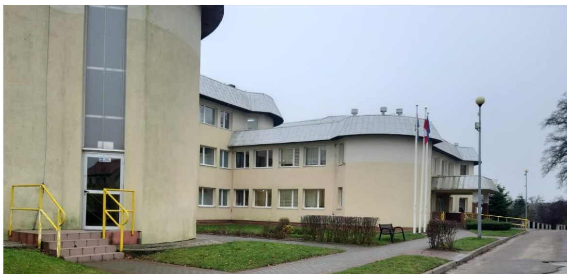
Figure 6-2. The school building's front facade
